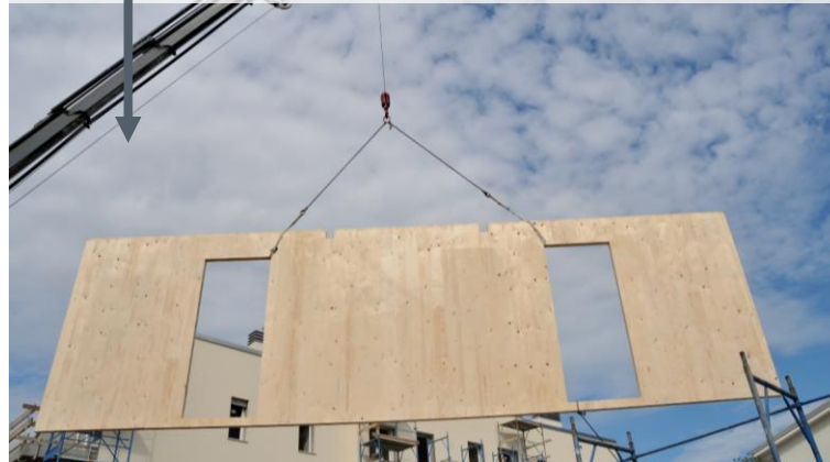
Shift to pre-fabricated building elements
